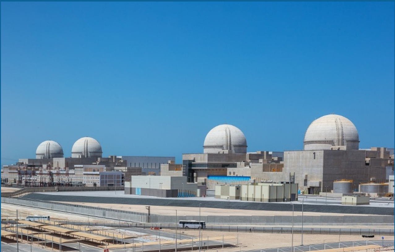
BARAKAH NUCLEAR POWER PLANT, UNITED ARAB EMIRATES
