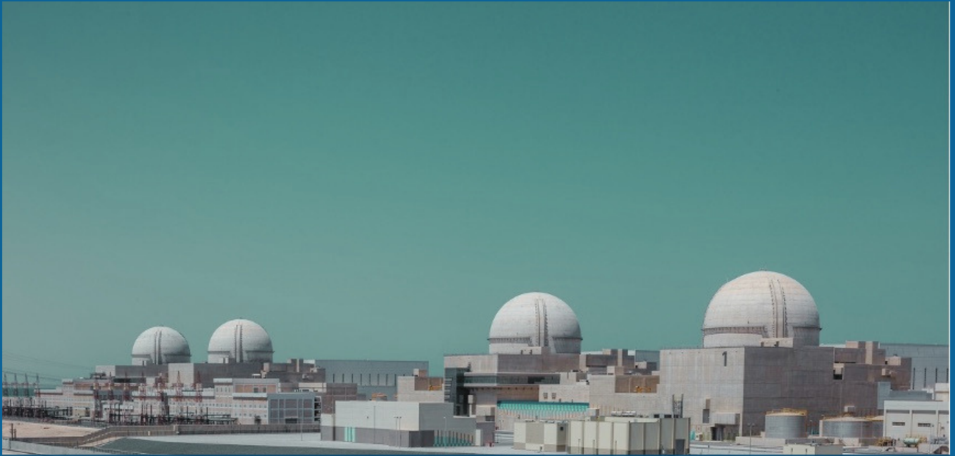
BARAKAH NUCLEAR POWER PLANT, UNITED ARAB EMIRATES
